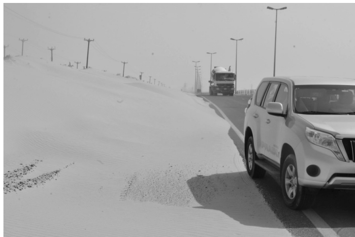
Figure 1(c). Sand encroaching on AlWafra-AlZoor Road (Author's camera, August 2018).
