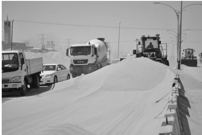
Figure 1(b). Partially closed lanes of AlWafra-Mena Abdallah Road (Author's camera, August 2018).
