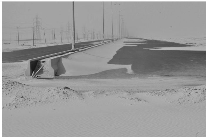
Figure 3(c). Roadside barriers (Author's camera, Aug 2018).
