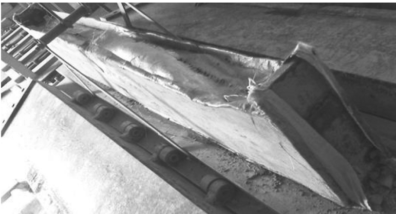
Fig. 2. Clay beam enveloped with Propylene fabric sheet during casting.
