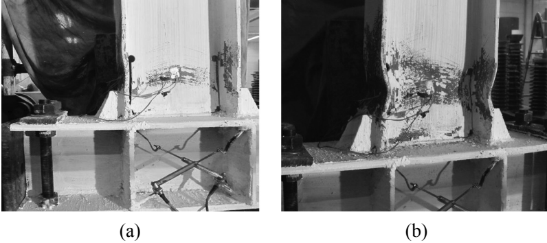
Fig. 15. Yield of beam flange and web & beam flange buckling
