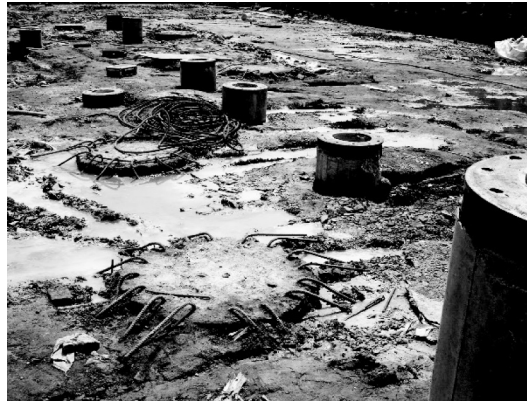
(a) PHC pipe piles and bored piles
