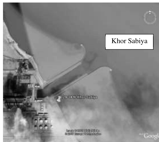
Fig. 5. Sabiya power plant intake structure in Khor Sabiya with sedimentation problem (Source: Google Earth).
