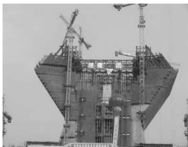
Fig. 8. The construction stage 6 in the practical project.
