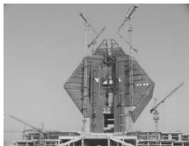
Fig. 9. The construction stage 9 in the practical project.
