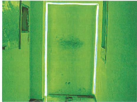
**Fig. 3.** Apartment door after installation of fire indicator lighting
