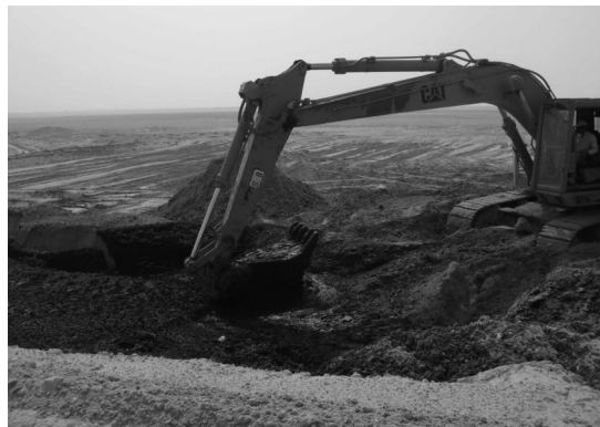
Fig. 3. Extraction of sludge by backhaul Truck.
