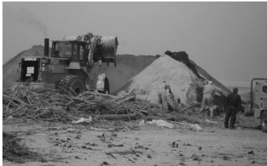
Fig. 5. Enhancement of anaerobic bacteria growth by adding nutrient (plants).
