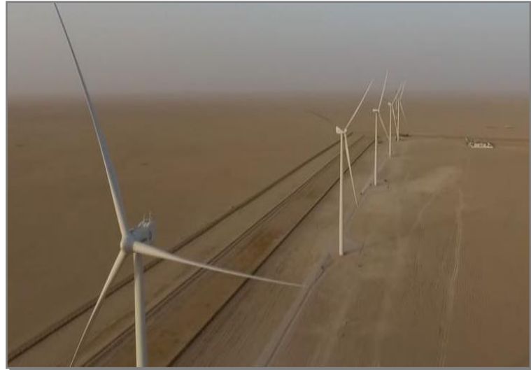
Fig.4. Wind turbine generators for Shagaya phase I.
