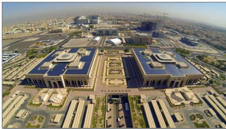
Fig.7. An aerial view of the MEWR and MPW rooftop PV systems.
