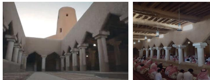
Figure 8. ‘‘Alsarha’’ the open courtyard as it was (left), and covered after rehabilitation in 2015 (right)
