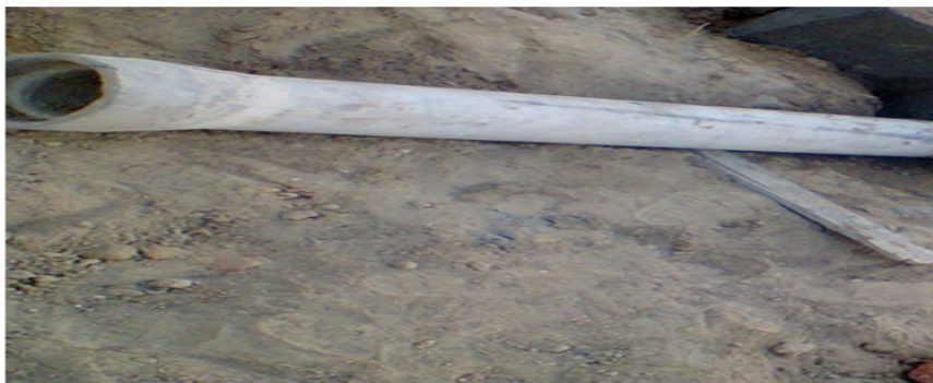
Figure 4. Pipe for Digestate
