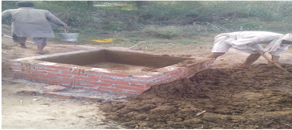
Figure 3. Construction of mixing tank
