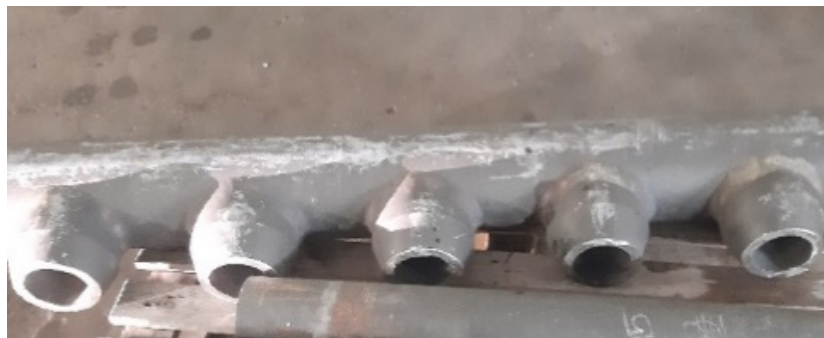
Figure 1. Outlet manifold bottom header.
