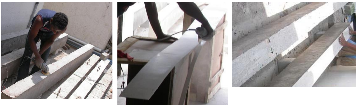
Figure 4. Process of grinding, cutting and adhering to beam
