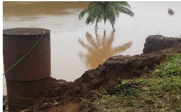
Figure 2 Depicts the open well damaged due to flood
