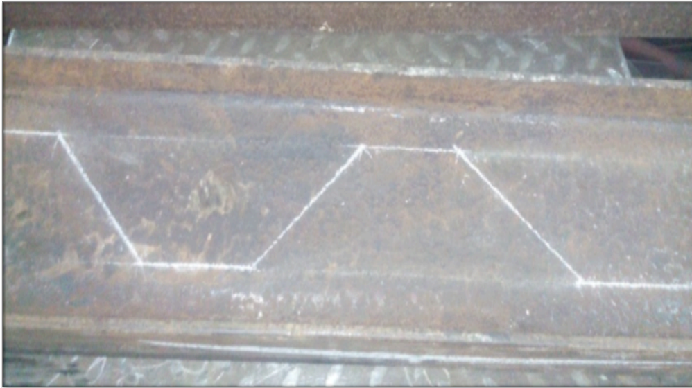
Figure 5 Marking of ISMB-200 section for castellation
