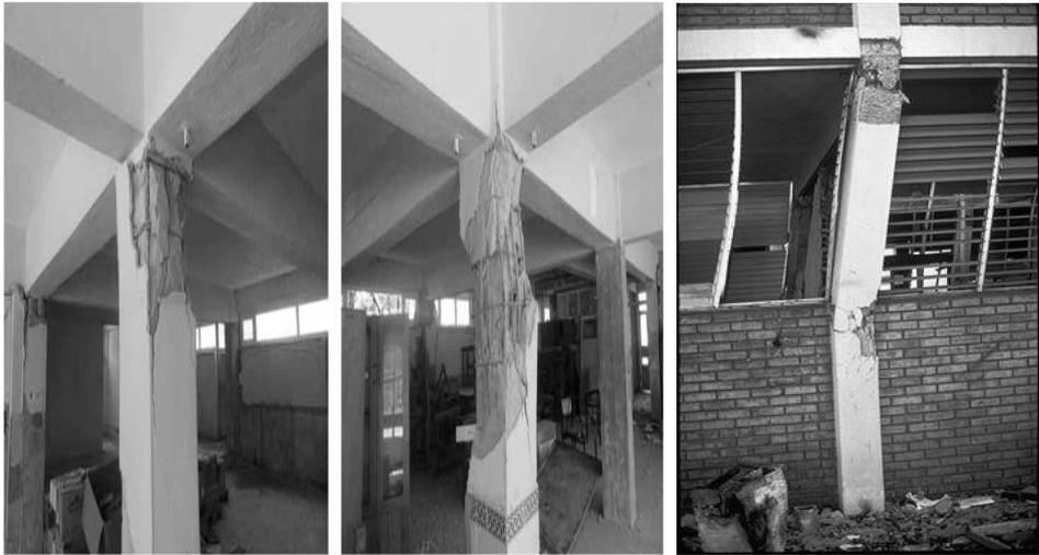
Fig. 12. Columns failure in a building with strong beams and weak columns.
