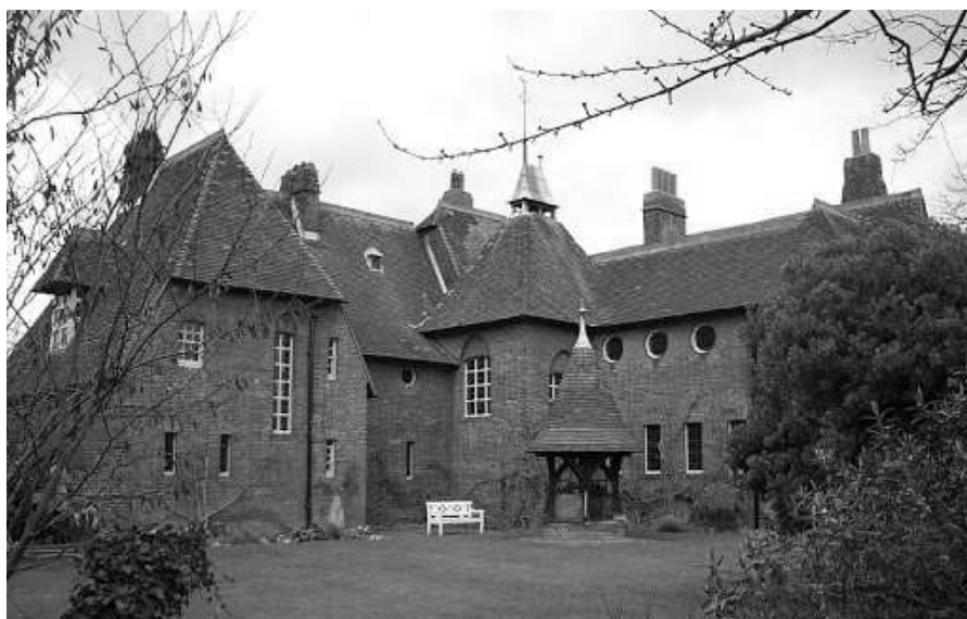
Figure 6. Red House by William Morris and Philip Webb, Bexleyheath, England ( https://smarthistory.org/william-morris-and-philip-webb-red-house/ ).
