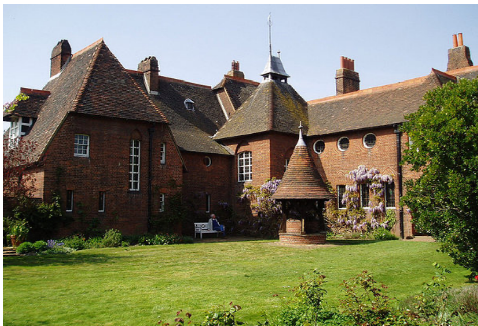
Figure 11. Red House by William Morris and Philip Webb, Bexleyheath, England. ( https://smarthistory.org/william-morris-and-philip-webb-red-house/ )
