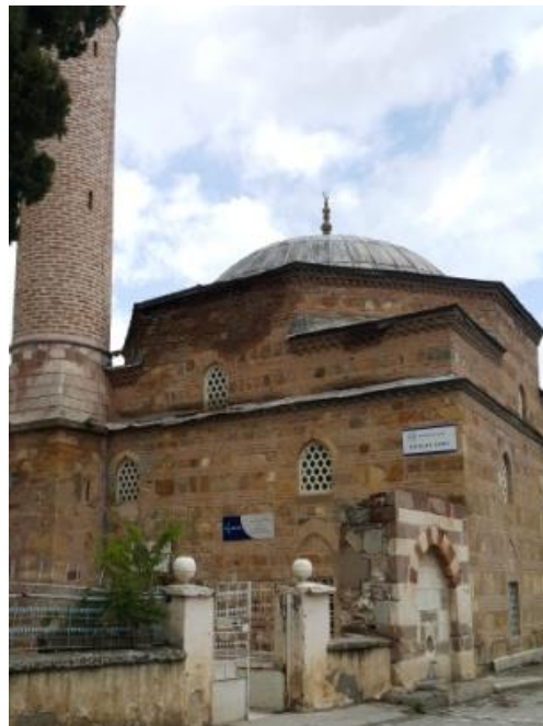
Figure 1. Sofular mosque General View.
