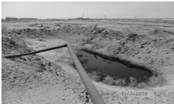
Figure 5. Wellhead pit photos show the present oil contamination.
