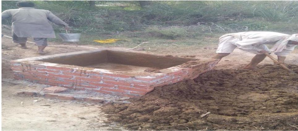
**Figure 3.** Construction of mixing tank
