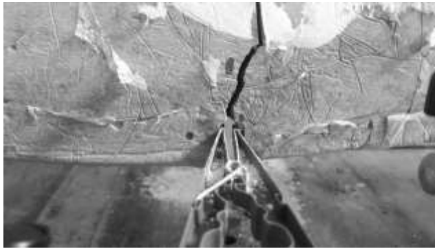
Fig. 10(b). Thick crack width of steel fibre reinforced concretes specimens (SHS-4).
