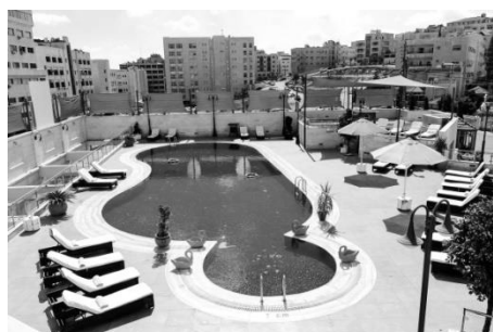
Figure 15. External pool in extension hotel building (designed by author).
