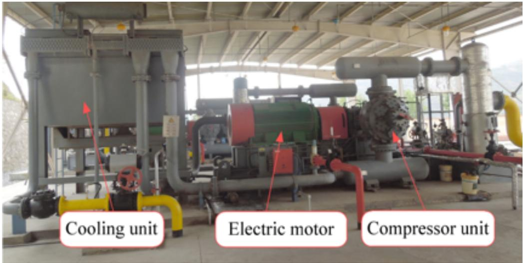
Fig. 3. Searable compressor driven by electric motor
