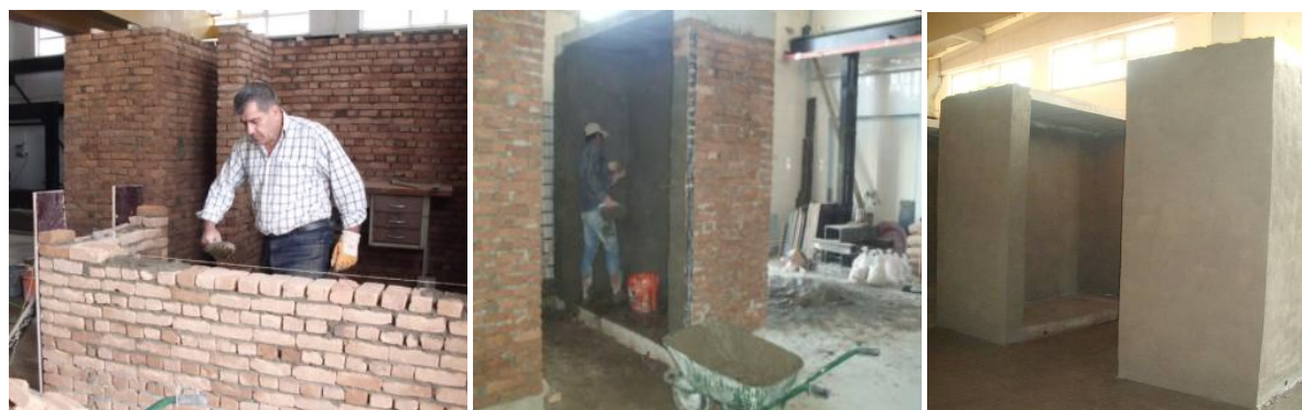
Figure 1. Brick wall samples
