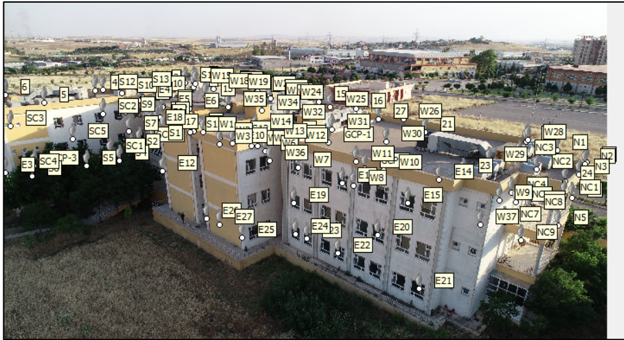
Figure 17. The east side control points; the control points of the west and south facades appear as well.
