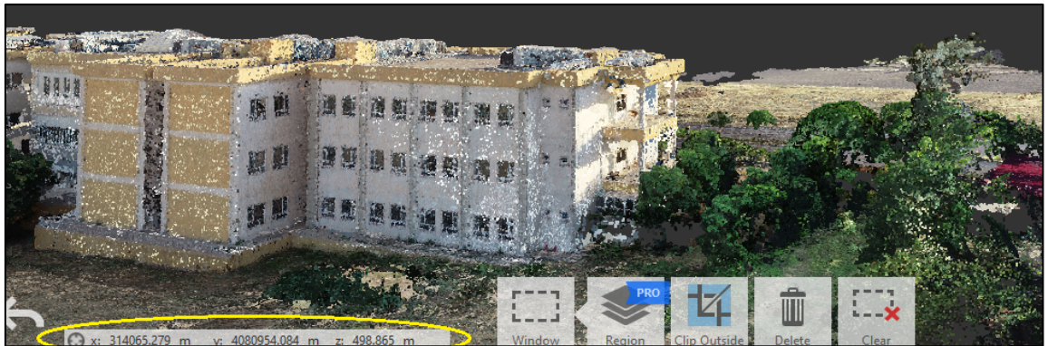
Figure 13. ReCap generated 3D model allowing to measure the coordinates of any point on the facades.
