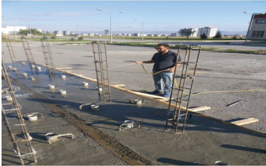
Figure 2. Curing of concrete foundation.
