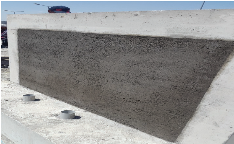
Figure 5. Application of plaster on the outer face of the infill wall.
