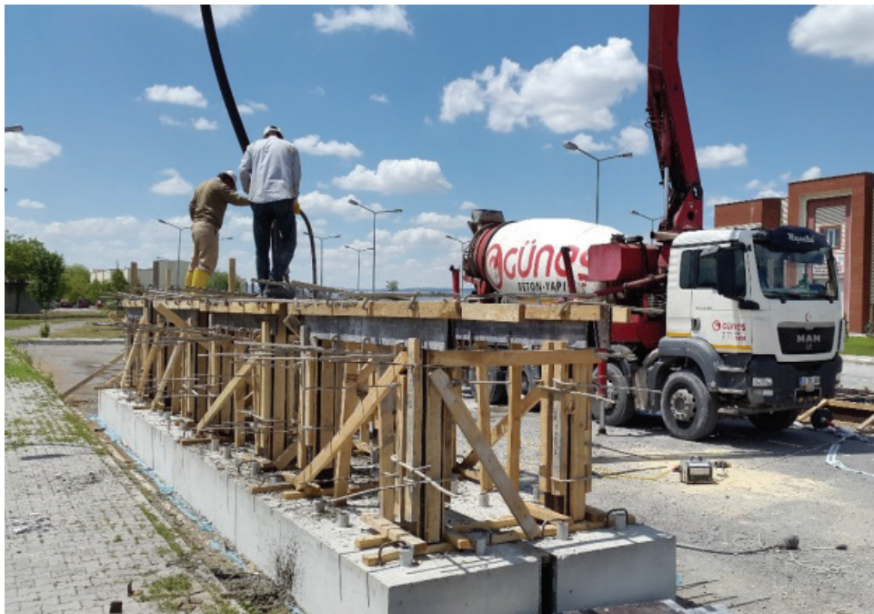
Figure 3. Pouring of frame concrete.
