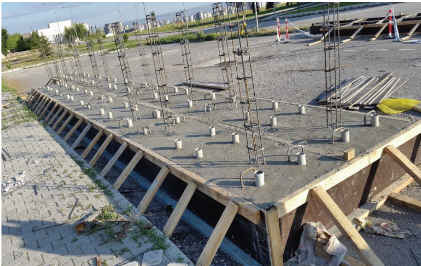
Figure 1. Foundation construction.
